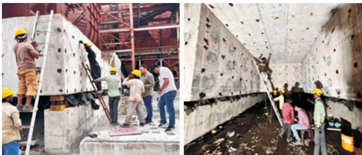
NDT studies in progress at site
