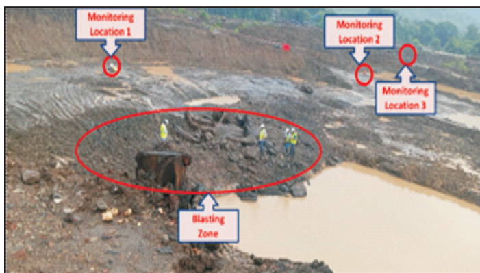
Trial blasting at lower reservoir in progress
