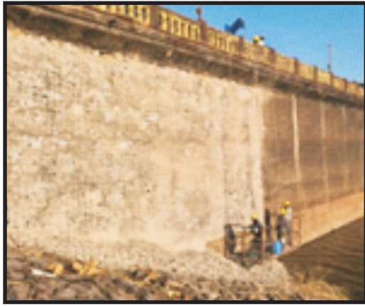
Chipping of gunitting in progress & chipped portion of U/s surface
