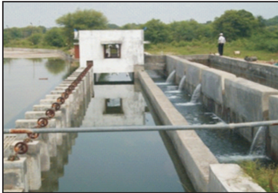
(A) ATG room with radial gates coupled to gate shaft along with supply & return channel (B) ATG setup in control room
