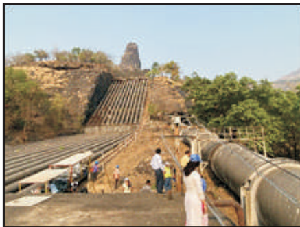
Panoramic View of Penstock Lines
