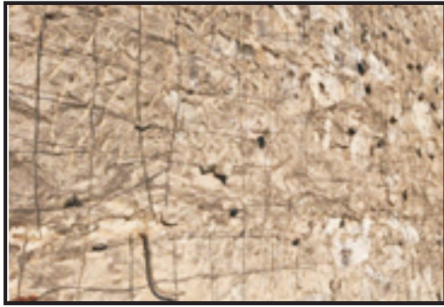
Chipping of gunitting in progress & chipped portion of U/s surface
