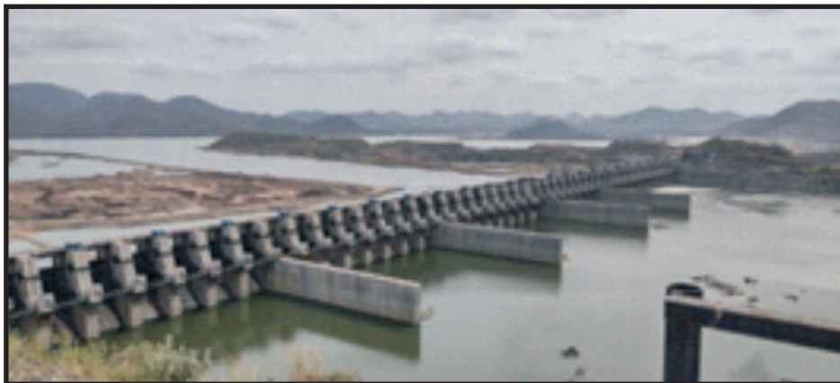
Panoramic view of Polavaram dam, Andhra Pradesh
